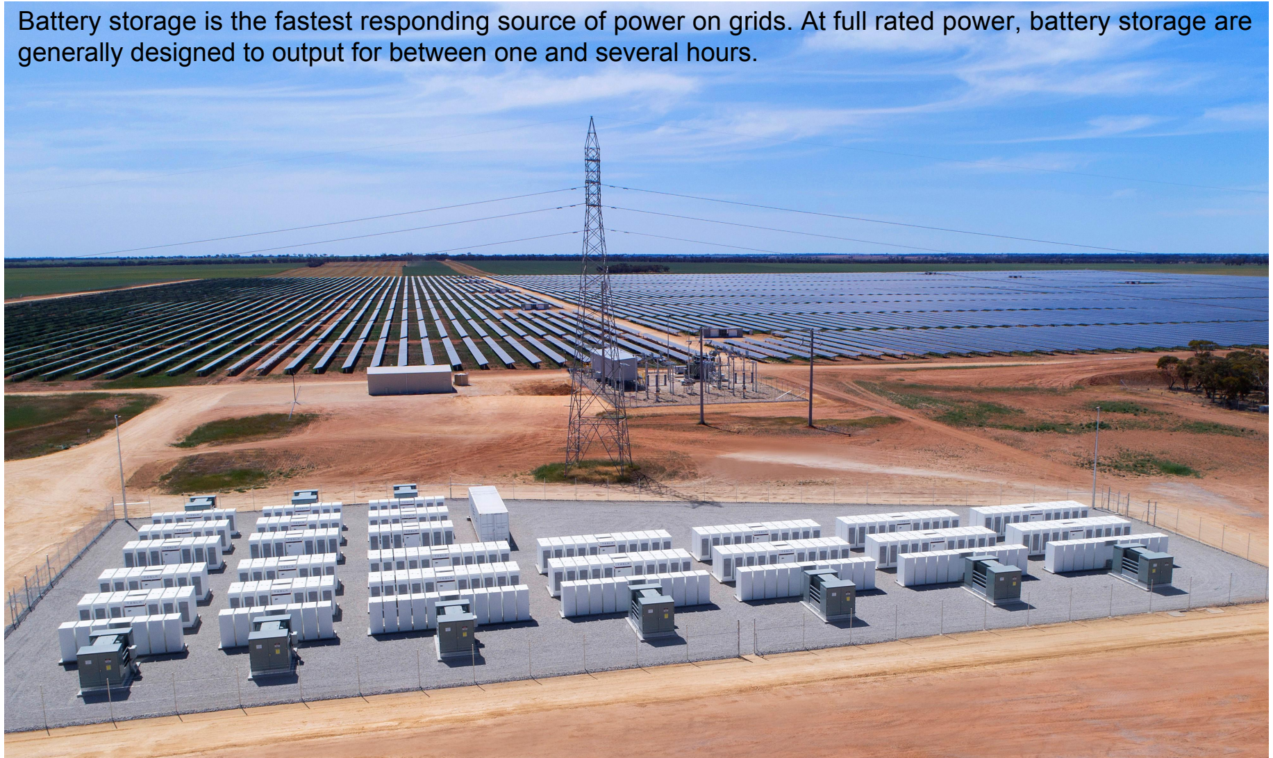
30 megawatt (MW) / 30 megawatt-hour (MWh) large-scale, grid-connected battery located at the Ballarat Area Terminal Station (BATS), Victoria, Australia.
