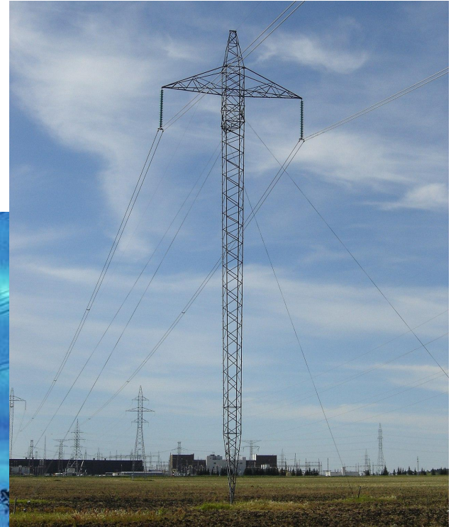
HVDC tower, Nelson River Bipole adjacent to Dorsey Converter Station, Canada
